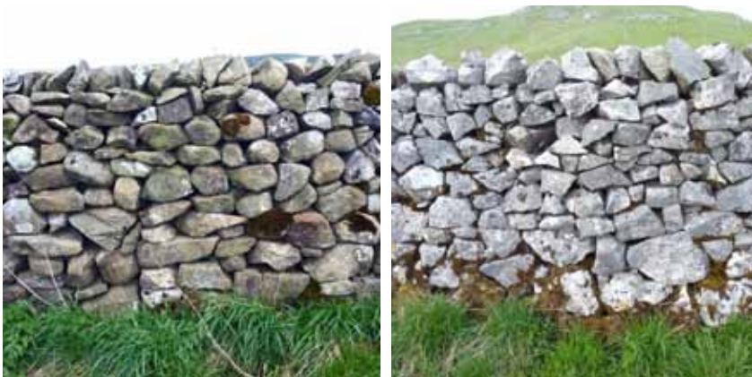
Left: a gritstone wall made from rounded boulders cleared from the fields Right: a limestone wall made from angular quarried rock © Tony Stephens
