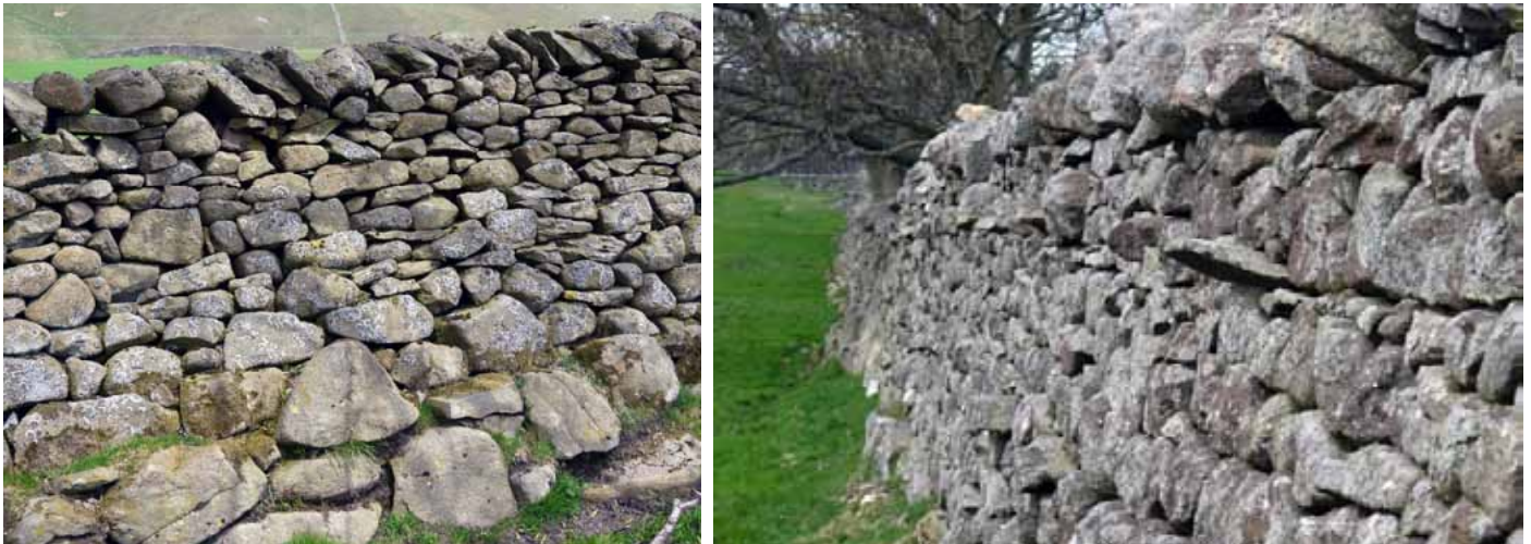
Left: the ancient wall round Newfield Right: A line of 'throughs' protrude from the post-1800 wall © Tony Stephens
